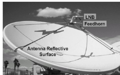
Fig. 2 Components of a Digital Satellite Dish.
